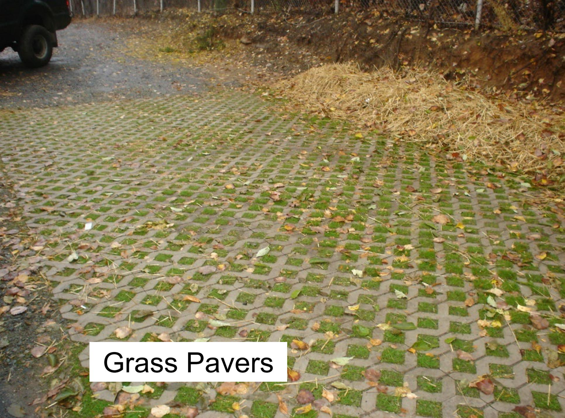
A photograph showing a driveway paved with interlocking concrete grass pavers. The pavers are arranged in a grid pattern, with green grass growing through the openings. The driveway is covered with fallen autumn leaves and some dry grass. In the background, there is a chain-link fence and a dark vehicle parked on the left. The overall scene is outdoors in an autumn setting.
